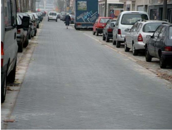
Fig. 4 Separate parking lanes at the Leien of Antwerp with photocatalytic pavement blocks
