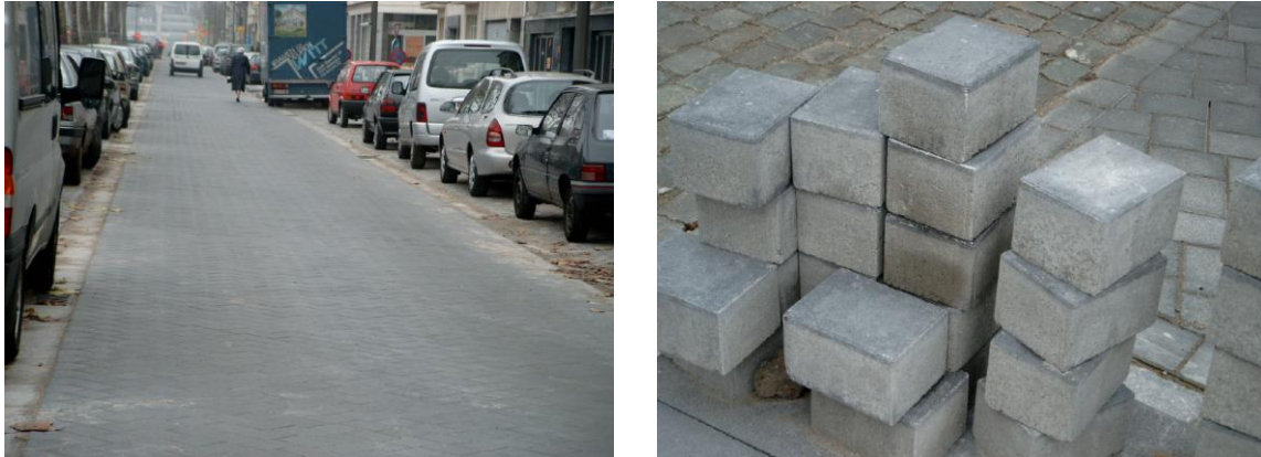
Figure 2 Separate parking lanes at the Leien of Antwerp with photocatalytic pavement blocks
